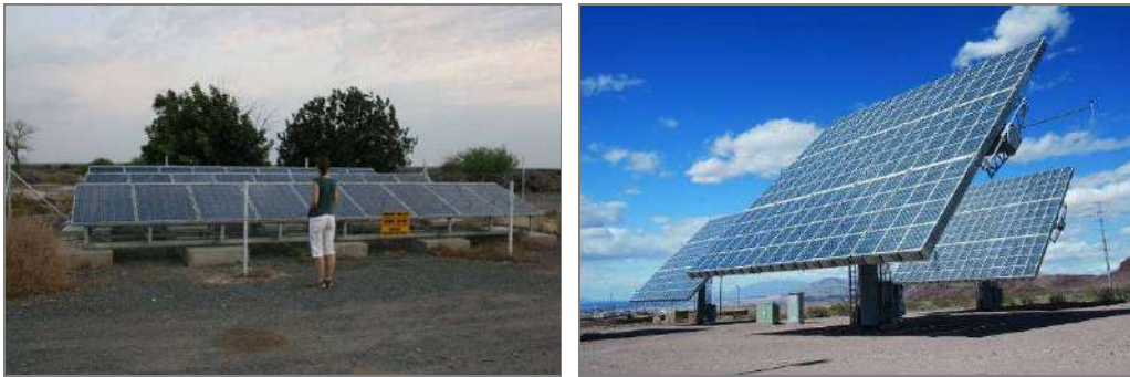
Figure 2.8 Photovoltaic solar cells (left) 24 and a CPV system (right) 25 were considered for the proposed PV plant
