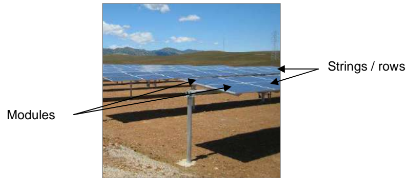
Figure 2.3 Typical layout of panel structures
