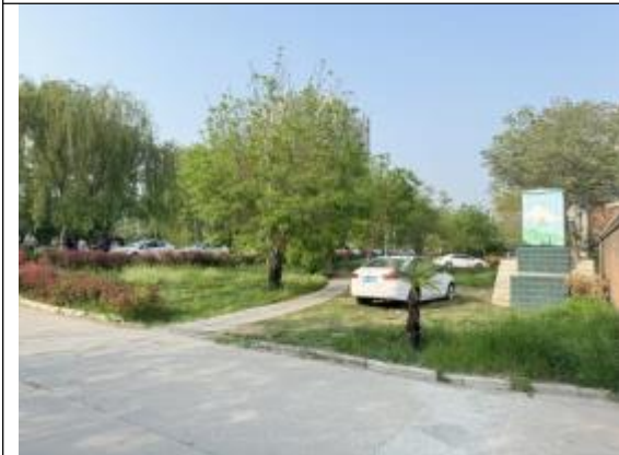
Surrounding environment of Xiangyang storm water pump station
