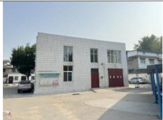
Xiangyang storm water pump station
