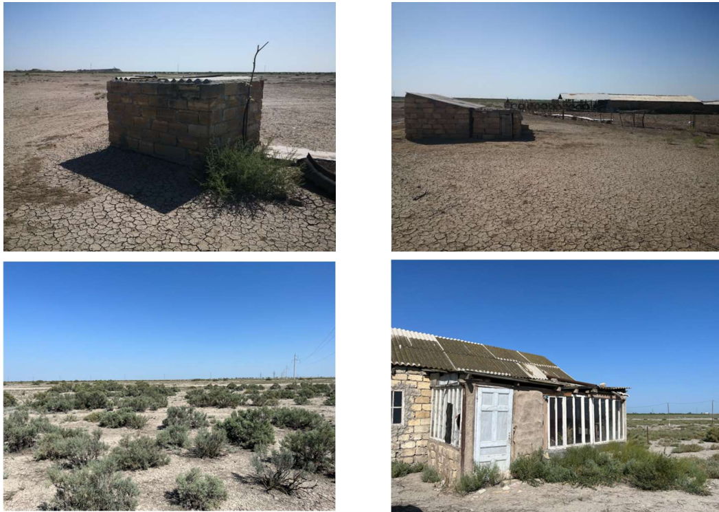
Figure 3-2 General Site Conditions and Existing Structures
