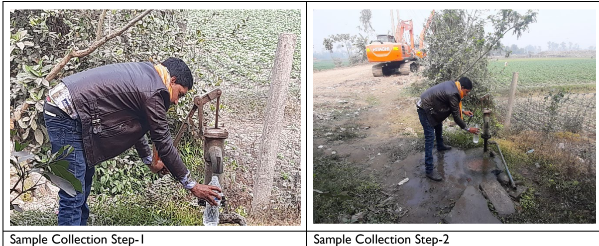
Figure 4.19 Ground water sampling pictures of RpCC landfill site tube well
