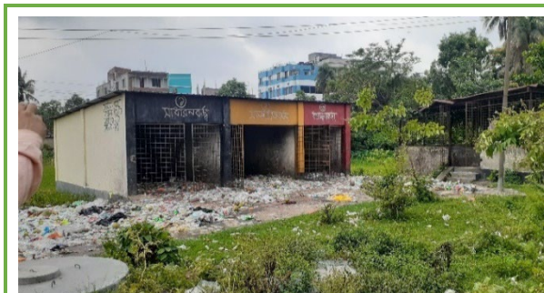
Example of secondary transfer station for waste collection
