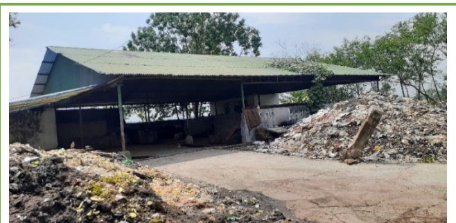
Example of secondary transfer station
