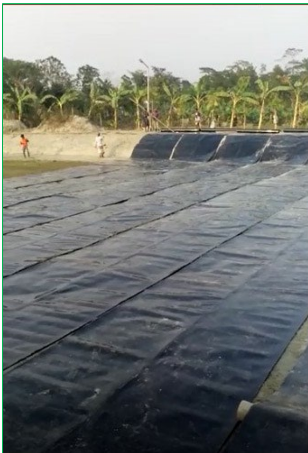
Figure 3-34: 1.5 mm thick HDPE Liner on top of the Clay Layer shall be used to manage leachate
