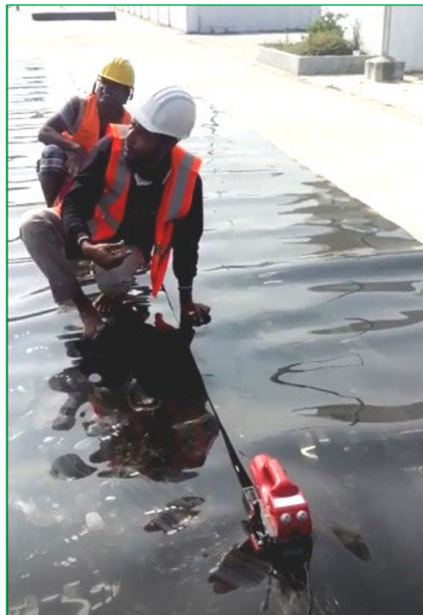
Figure 3-34: 1.5 mm thick HDPE Liner on top of the Clay Layer shall be used to manage leachate
