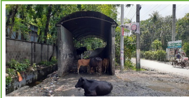
Secondary Waste Storage in Dilapidated Condition
