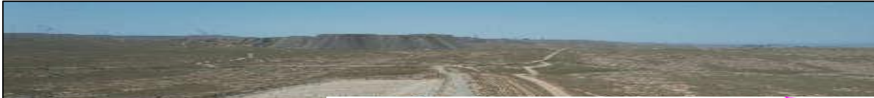
A.3. Construction site – general view
