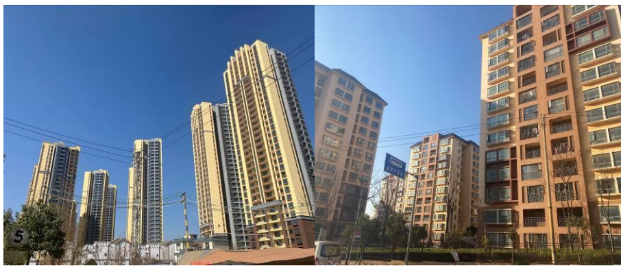
Figure E-1 Photos of Resettlement Residential Areas
