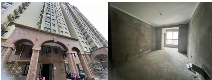
Figure 5-5 Exterior and Interior of Building 11 of Chunjiang Garden
