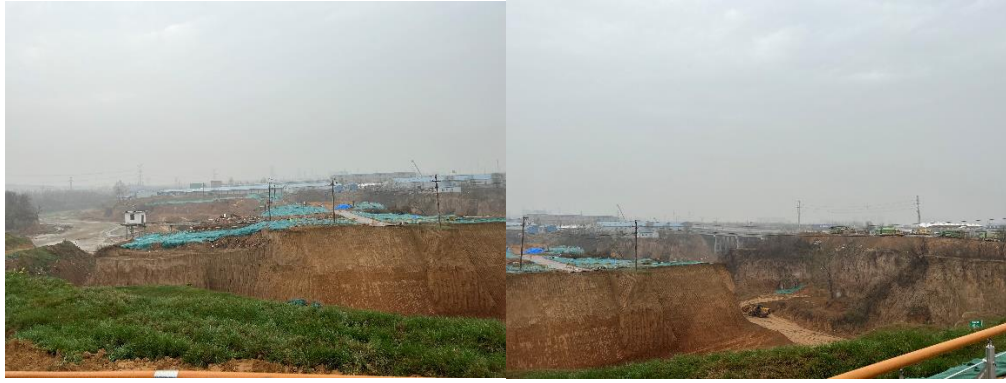
Figure 1-4 Construction of the Guojiazui Reservoir
