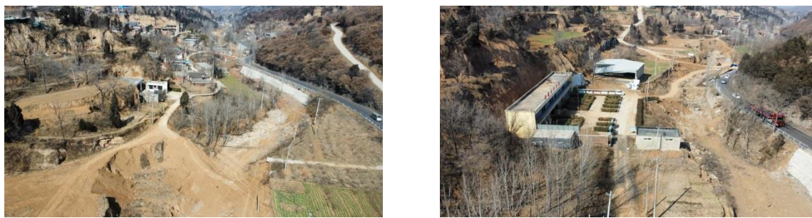
Figure 4-4 Current situation of some flood-damaged roads
