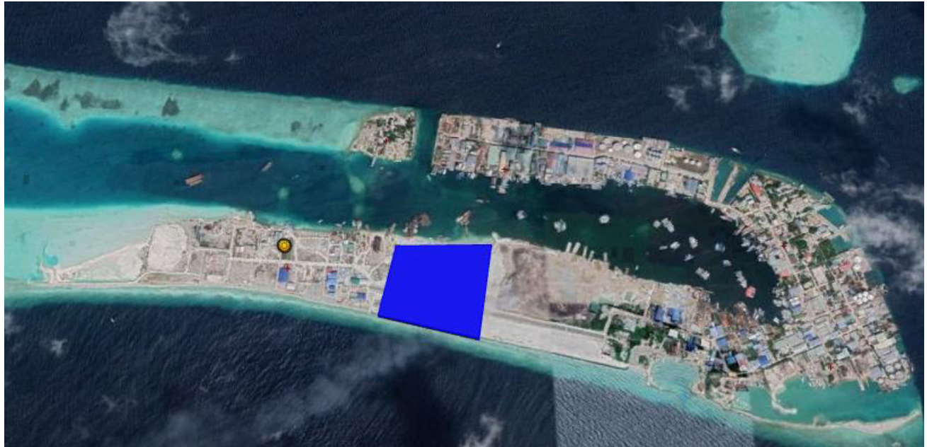
Figure 21: Building Area of WTE Plant
