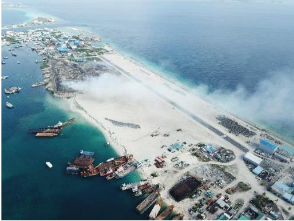
Figure 7: areal picture of reclaimed area for WtE Facility
