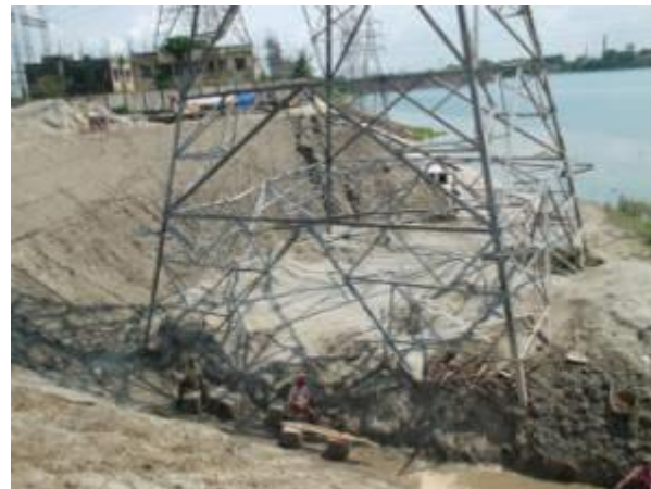
Figure 3.18: Placing tower on its foundation
