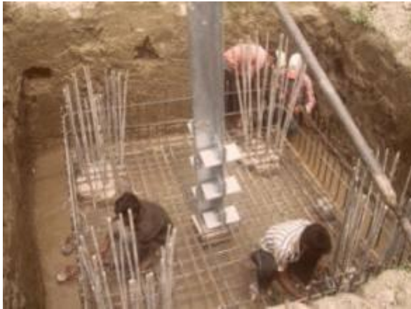
Figure 3.15: Stripping the tower footing with steel
