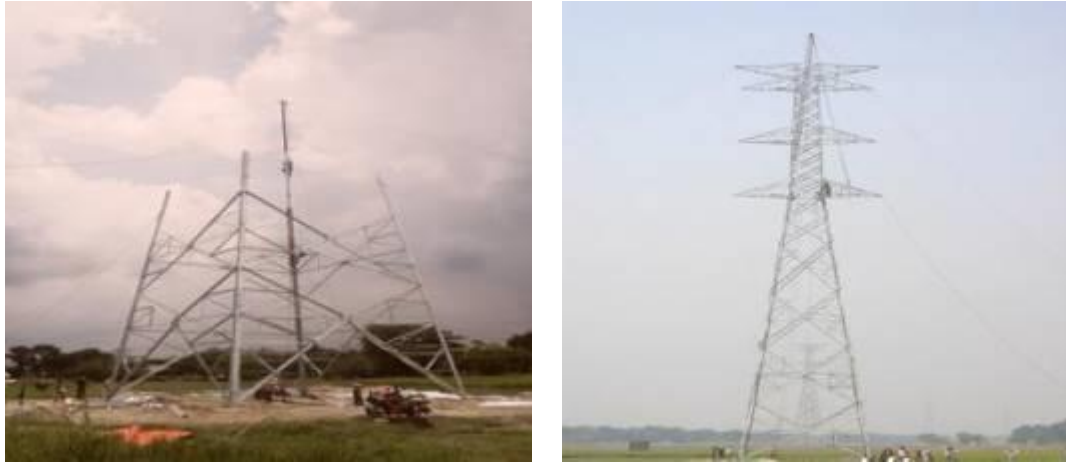
Figure 3.19: Tower erection works
