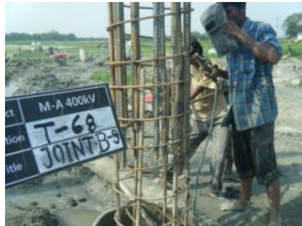
Figure 3.12: Welding of reinforcements
