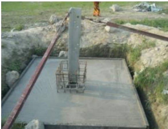
Figure 3.17: Casting concrete cement into tower foundation
