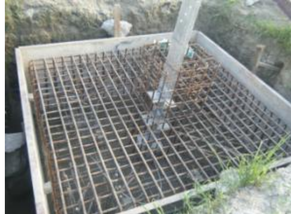
Figure 3.16: Providing detail reinforcements
